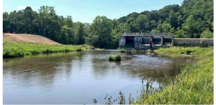
Late July view of dam construction Photo by Nick Schmit
