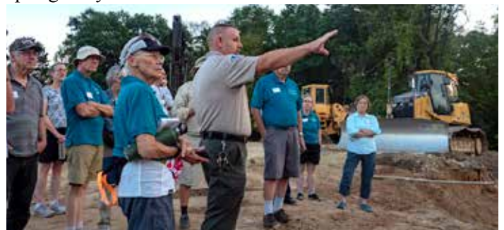
Park Superintendent, Aaron Mason, points out construction highlights. Photo by Dave Thofern
