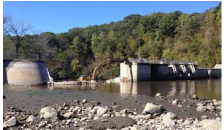
Excavator works to breach Willow Falls Dam
